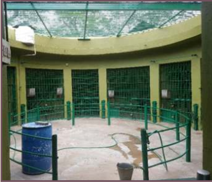
RENOVATION OF CHIMPANZEE HOUSE
